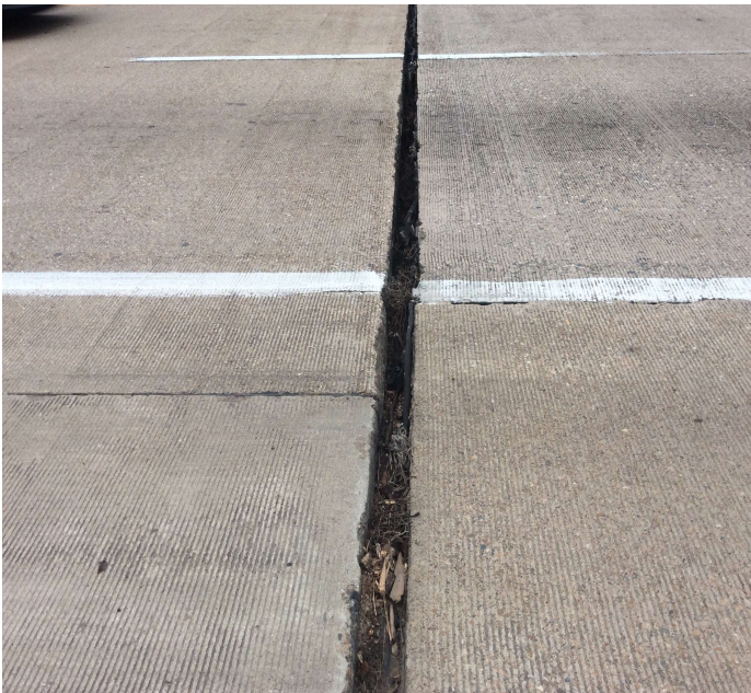
PHOTO 7 Description JOINT MATERIAL MISSING END OF BRIDGE
