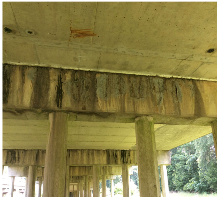
PHOTO 6 Description BT 10 spalls with rebar exposed 10 LF Area has some paint
