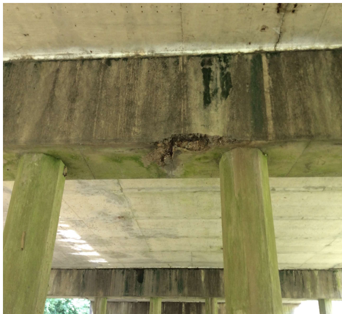
PHOTO 19 Description Bent 23 spall bottom of cap rebar exposed.
