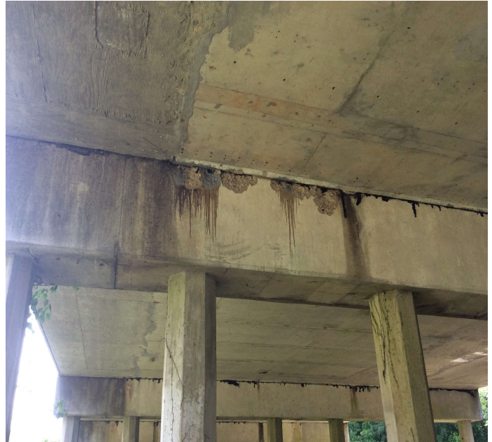
PHOTO 17 Description Bent 22 spall top of cap west face
