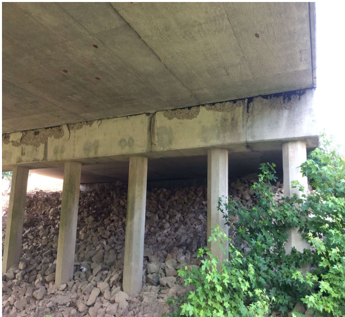
PHOTO 1 Description BT 2 cap spalls 18 LF
