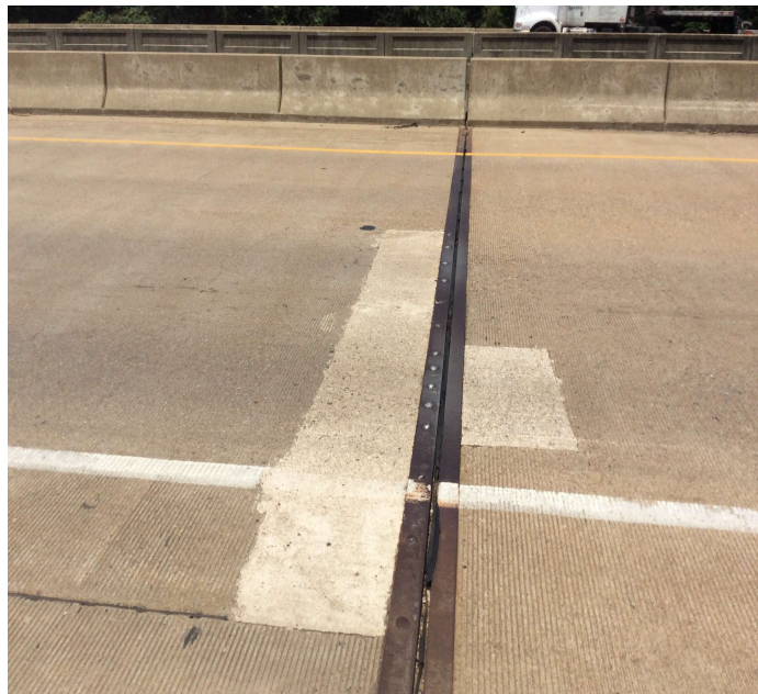
PHOTO 4 Description Bent 15 joint missing material,leaking
