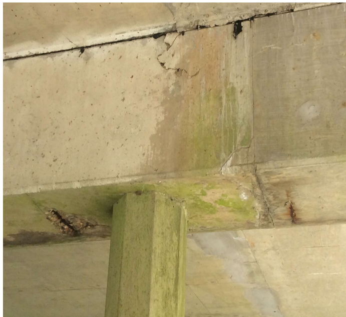
PHOTO 20 Description Bent 24 spalls, spalls with rebar exposed, and delams.
