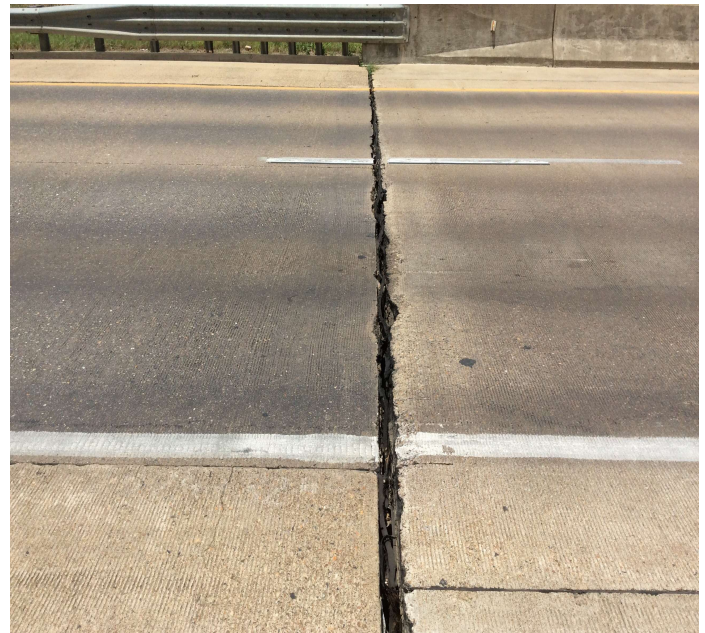
PHOTO 5 Description Bent 1 missing material 2 1/2"
