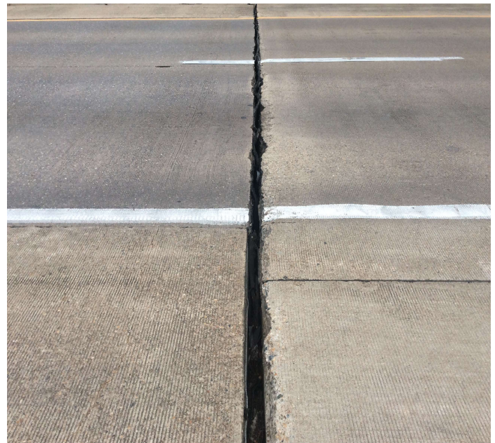
PHOTO 6 Description JOINT MATERIAL MISSING BEGINNING OF BRIDGE.
