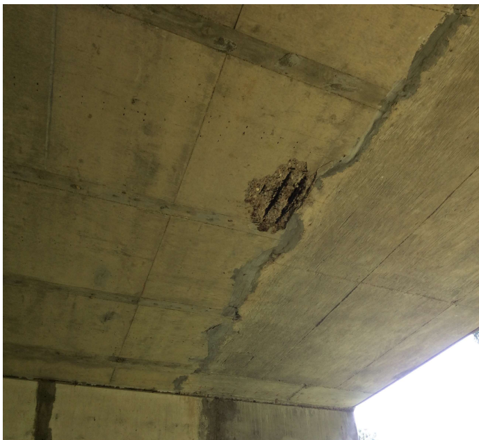
PHOTO 7 Description Span 14 spall rebar exposed 4 sq ft section loss to rebar.
