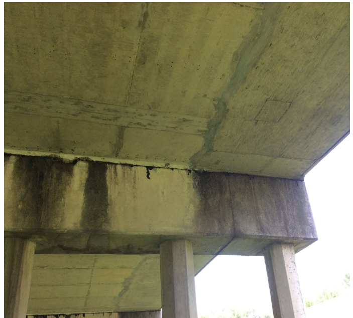
PHOTO 5 Description BT 9 spall at pile 2 for 2 LF
