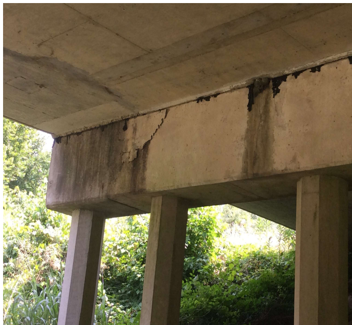
PHOTO 21 Description Bent 25 spalls and delams.
