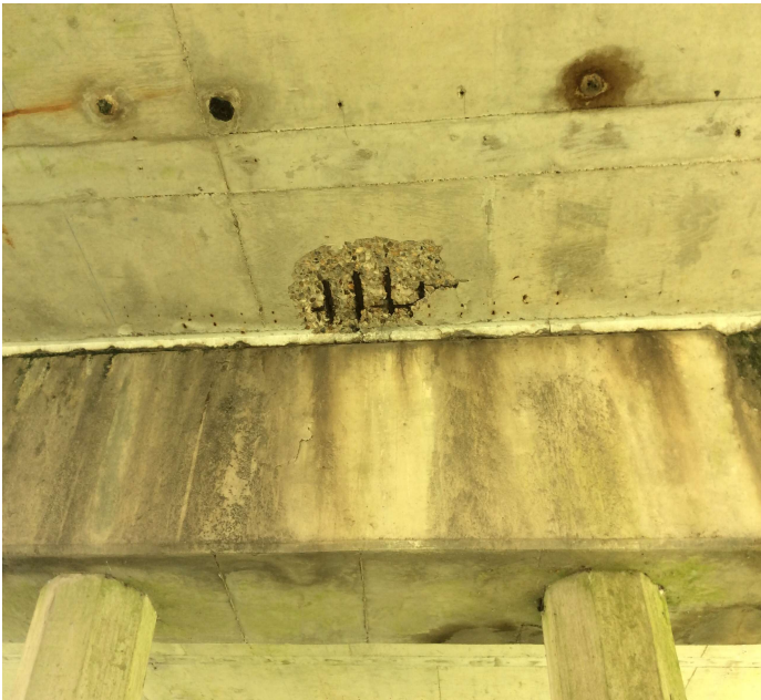
PHOTO 4 Description SPAN #8 AT BENT # 9 BETWEEN PILES 4 & 5 SPALL W/REBAR EXPOSED IN SOFFIT 3 sq ft
