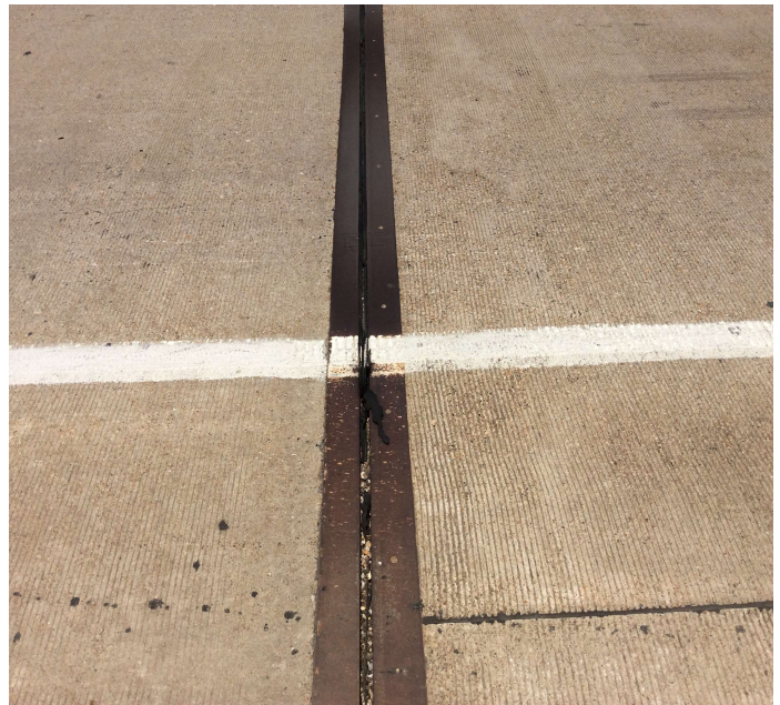
PHOTO 2 Description Bent 16 joint needs cleaned and refilled
