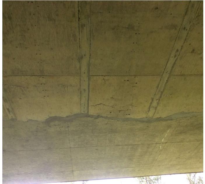
PHOTO 5 Description Delam bottom deck 4 sq ft Efflorescence also.
