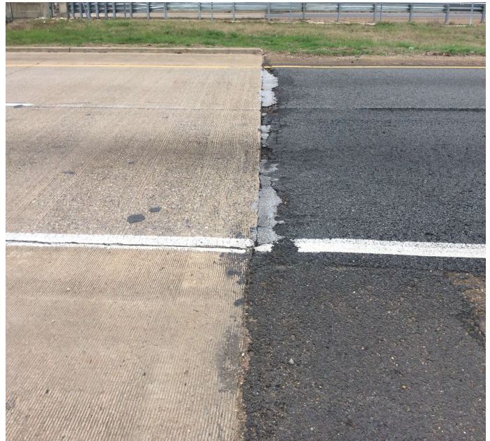
PHOTO 2 Description ASPHALT AT END OF APPROACH NEEDS REPAIR.
