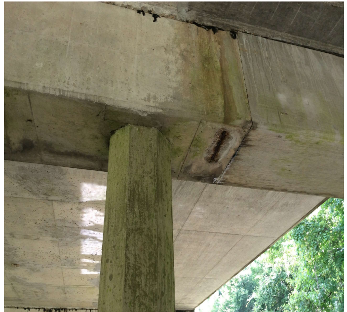
PHOTO 18 Description Bent 22 spall bottom of cap rebar exposed.
