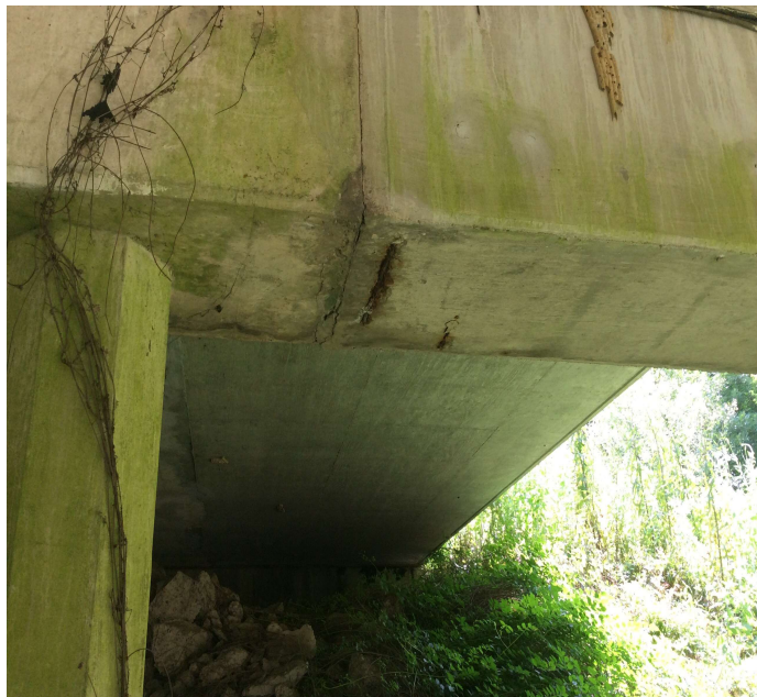
PHOTO 22 Description Bent 25 spall rebar exposed
