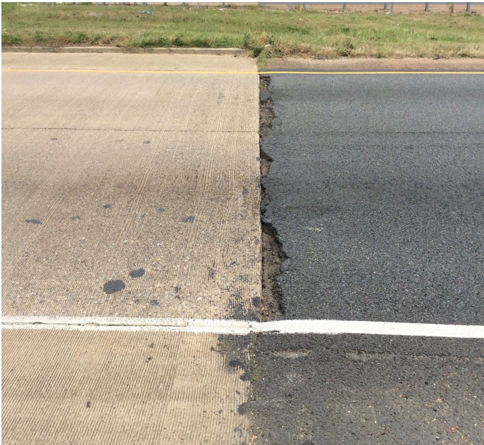
PHOTO 1 Description End of approach slab west bound lanes deep ruts and pot holes
