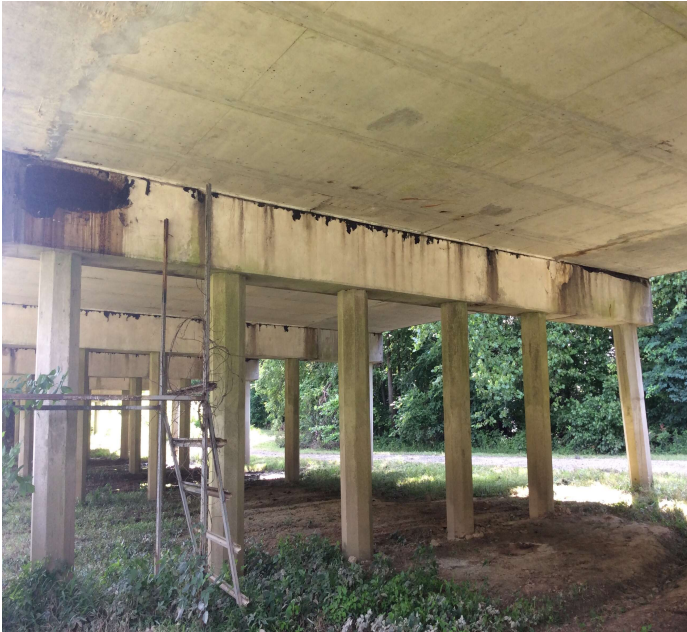
PHOTO 15 Description Bent 20 spall with rebar, and delams.
