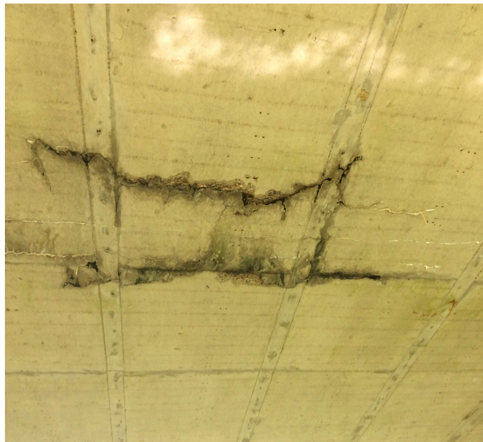
PHOTO 1 Description Lg delam 8'x 3' and spall 24 sq ft span 4 center bridge
