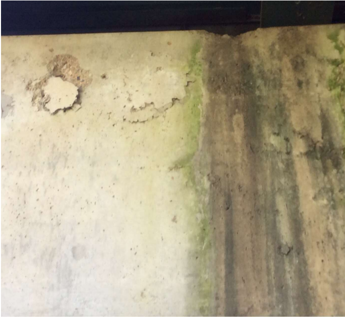
PHOTO 11 Description Delams at bent 16
