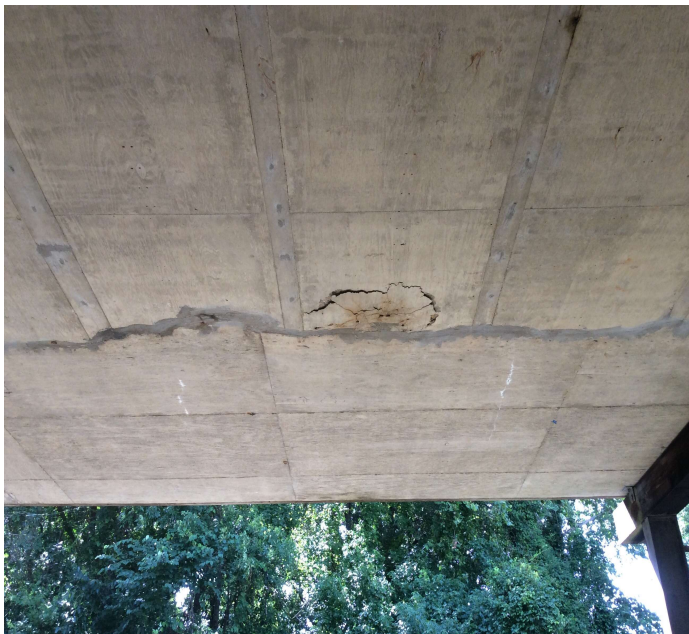
PHOTO 8 Description Span 18 delam
