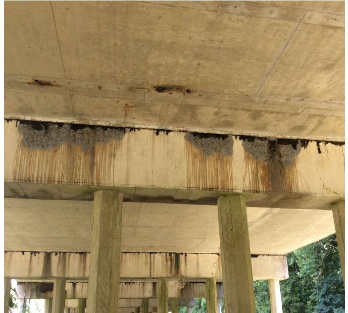
PHOTO 13 Description Bent 18 large spall west face
