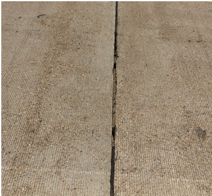
PHOTO 1 Description Construction joints need to be cleaned and refilled
