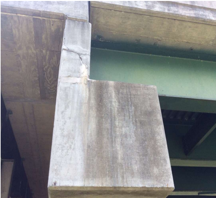
PHOTO 12 Description Crack in riser at bent 16
