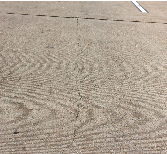
PHOTO 1 Description Span 27 deck cracks
