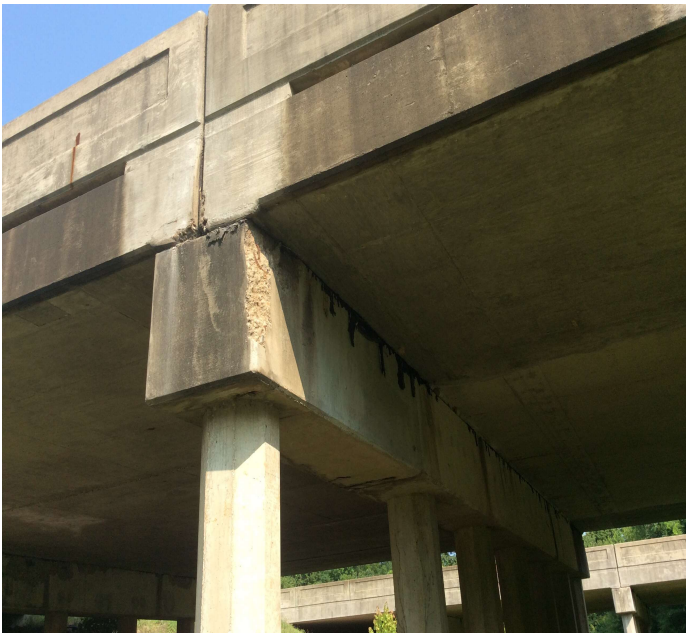
PHOTO 1 Description Bent 3 cap spall on rt and lt ends 3 LF
