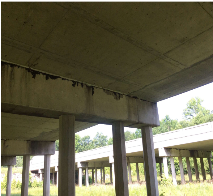
PHOTO 4 Description BT 7 cap spall 3 LF at pile 3
