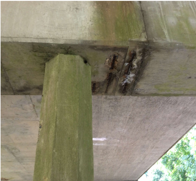
PHOTO 16 Description Bent 21 spall with rebar exposed
