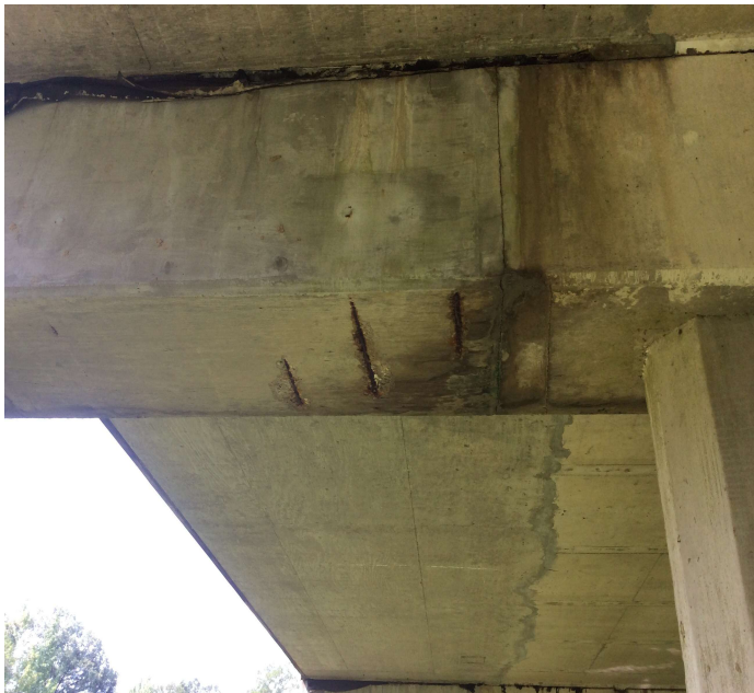
PHOTO 3 Description Bottom cap spall rebar exposed 2 LF Between pile 6 & 7
