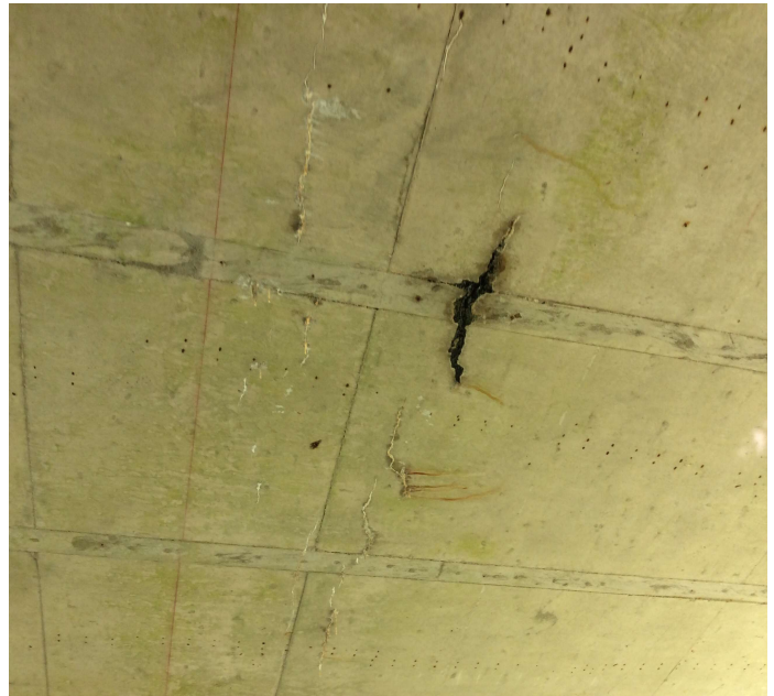
PHOTO 6 Description Span 12 efflorescence 40 sq ft white stain 2 sq ft black stain
